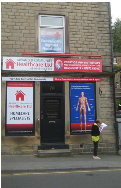
Large fascia and adverts covering three windows.
