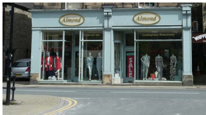
Example of reinstatement of historic-style shopfront.
